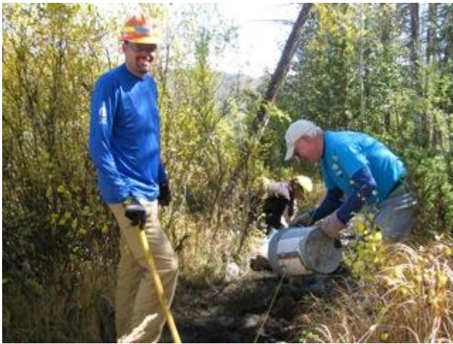
Ken and Pat building the AA Bar Barn Trail
